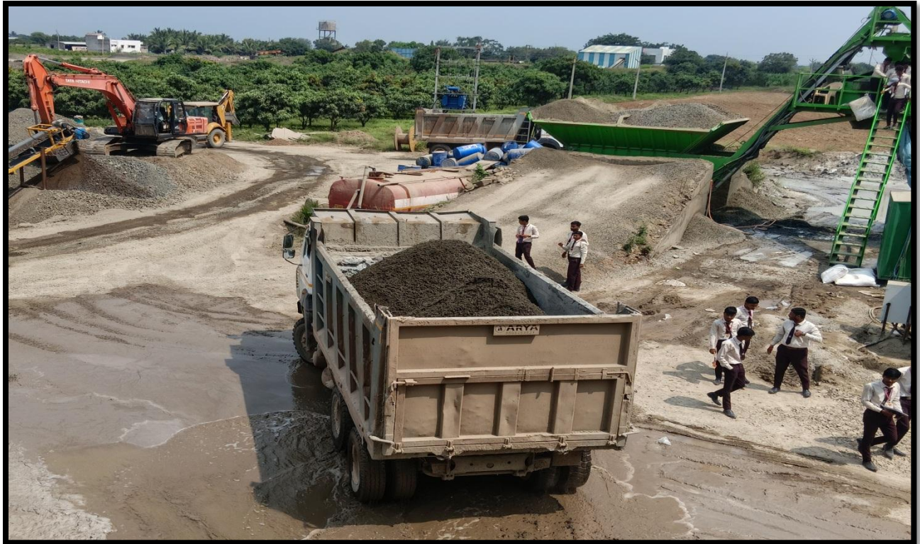
M10 CONCTRETE READY TO TRANSPORT NEAR BY SITE
